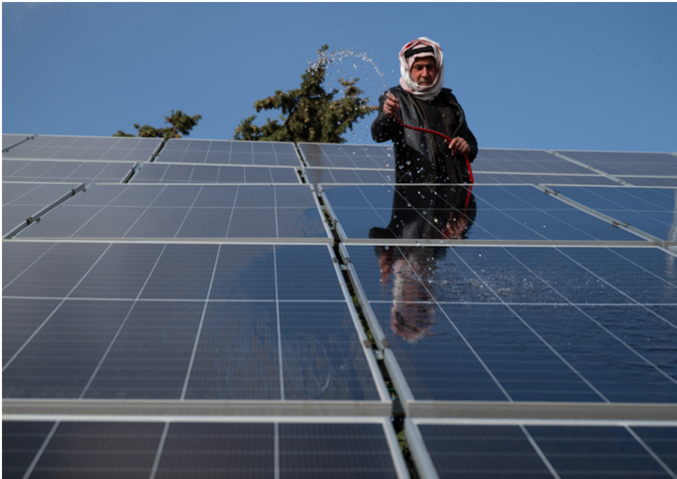
Solar panels installed at a borehole in rural Hama, Syria. Fawaz Alkhaled conducts routine cleaning to maintain system efficiency. Photo: Håvard Bjelland/Norwegian Church Aid
