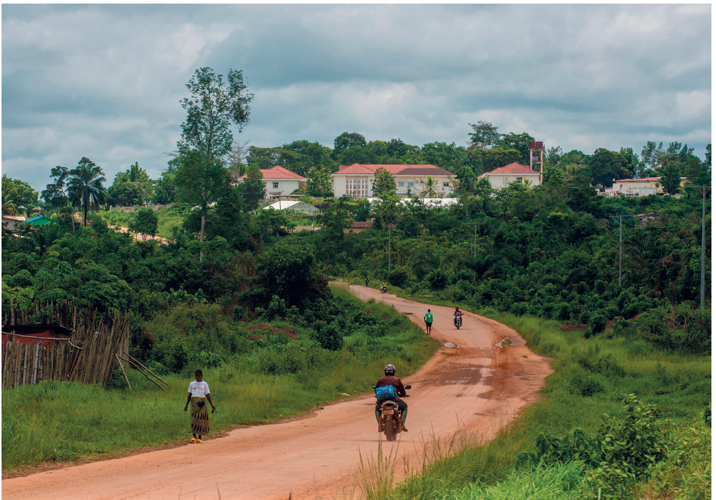
View of Jackson F Doe Regional Referral Hospital, Tappita from a distance.
